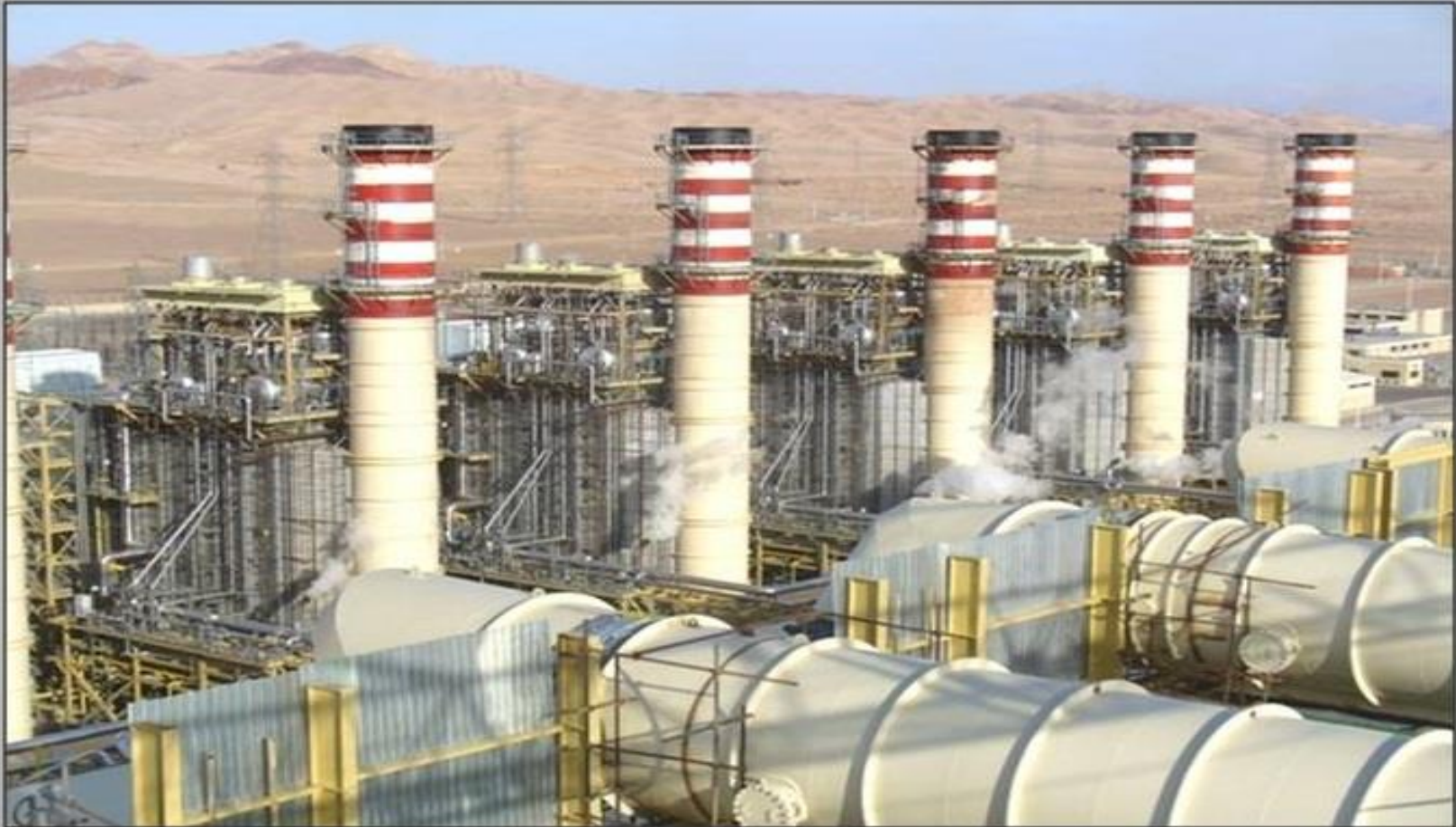
KERMAN combined cycle power plant
